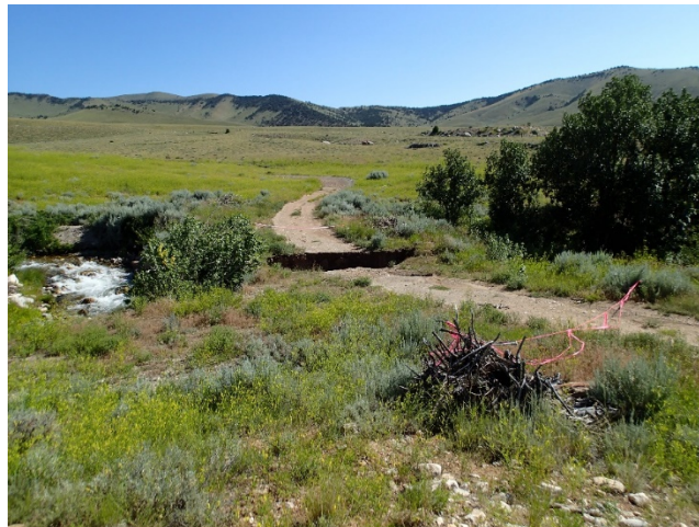
Figure 11: An undersized culvert on Line Creek (NFSR 123) did not pass flood flows during a storm event. The pipe was likely plugged by woody debris, forcing water over the road and carrying road fill downstream where it was eventually deposited into aquatic habitats. Fire consumed much of the watershed and a flood event also contributed to the failure of this stream crossing.
