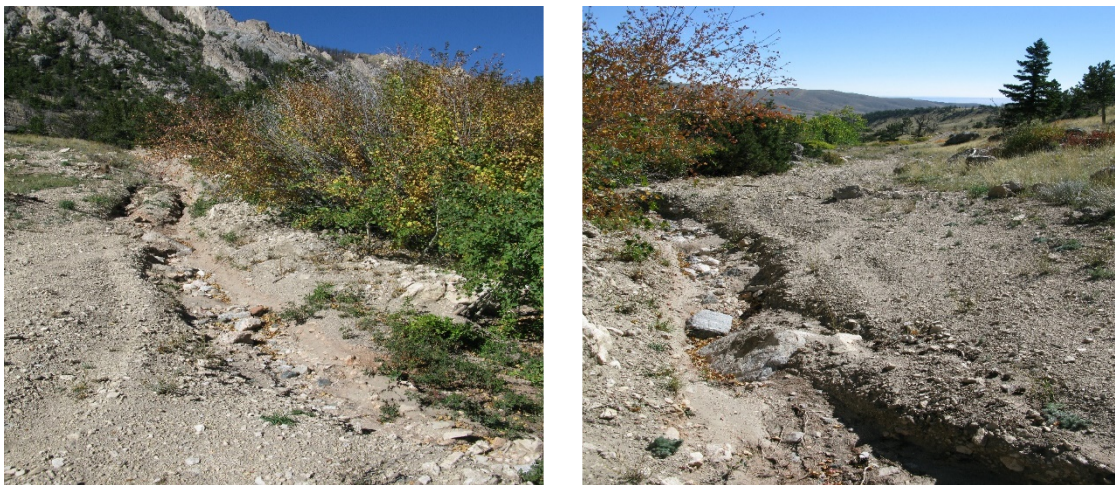
Figure 10: Roads (NFSR 123) that parallel riparian areas such as this road along Line Creek, capture sediment where it is diverted into the stream channel (hidden by woody vegetation).
