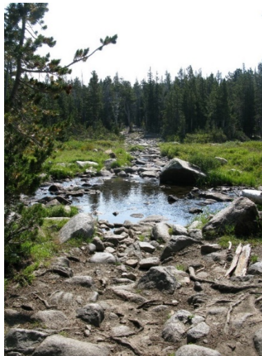
Figure 12: A low water crossing on the Christina Lake Road (NFSR 355). While aquatic organism passage is unimpeded at stream crossings such as this, low water crossings can become chronic sources of sediment inputs. Habitats at these types of crossings tend to be unnaturally wide, shallow, and generally provide poor fish habitat. This road would be converted to a motorized trail under Alternative 2.
