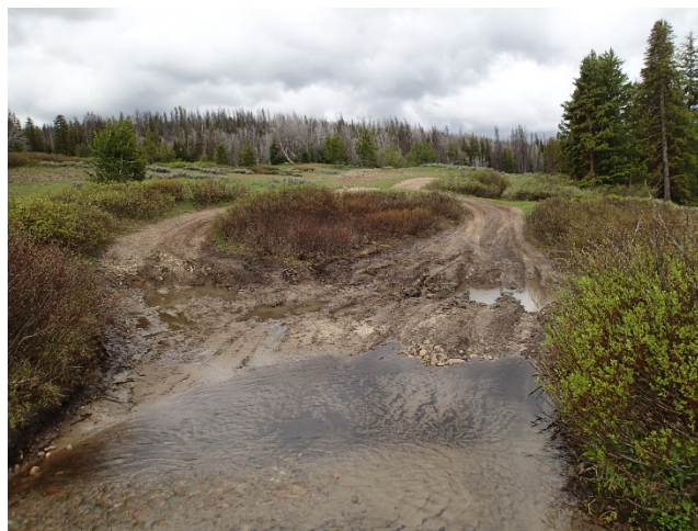
Figure 13: NFSR 534 intersects a wetland adjacent to Fish Lake. Difficult travel conditions lead to "pioneering" or the creation of new routes that, in time, can conditionally degrade to equally adverse condition. There are opportunities in travel management to relocate roads in high-risk areas such as this to more responsible locations (a reroute is proposed
