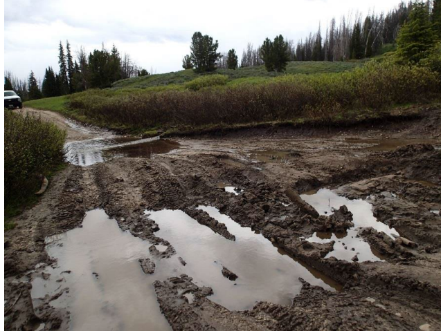
Figure 21: Alternative 3 would move this road uphill onto an adjacent bench. There is a high probability erosion into Fish Lake would be reduced and wetland habitats could be restored if Alternative 3 were selected.
